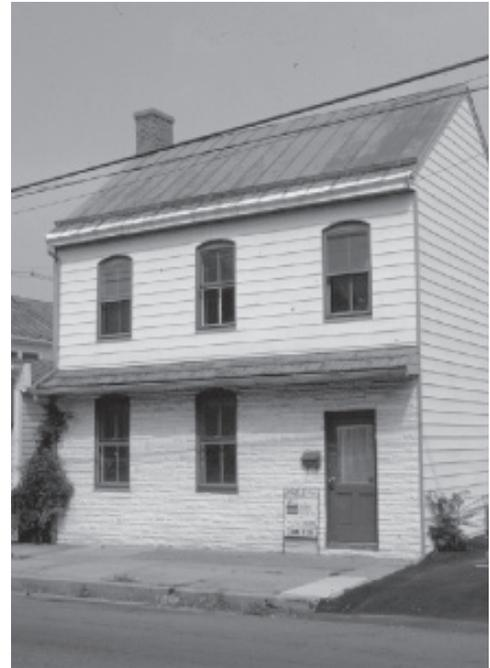
Frequently, the installation of artificial siding results in the removal of historic elements like brackets and porches.
