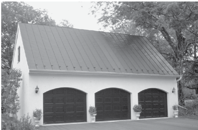
New garages can be designed with steep metal roofs and segmental arched openings to reinforce the historic character of the district.
