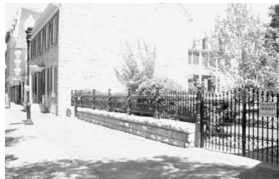
A combination of limestone base and a wrought iron fence creates an attractive and historic edge to the property.
