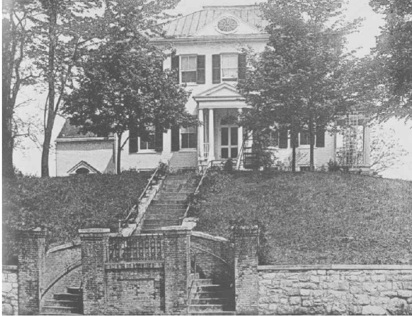
Steps leading to Conrad House were demolished to construct a parking lot in front of Judicial Center.
