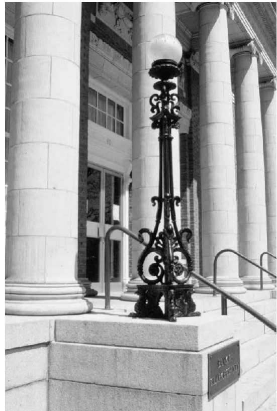
Historic light fixtures like this ornate example are an important site feature and should be preserved.
