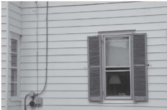
Artificial siding does not have the appearance or patina of real wood siding.
