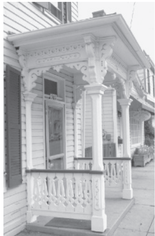
The elaborate design of this wooden porch is created with decorative brackets, posts, cornice pieces, and the cutout balustrade.
