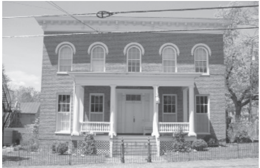
In this historic house the main cornice with brackets helps define the dwelling's Italianate style, while the classical cornice of the porch reveals that this element is a later change to the property.
