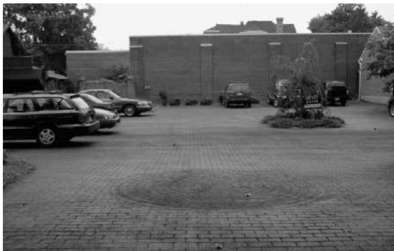
Distinctive brick paver patterns add character to the surface of this asphalt parking area.
