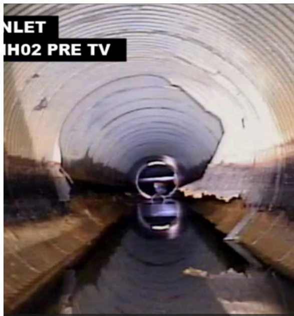
Culvert condition prior to lining.
