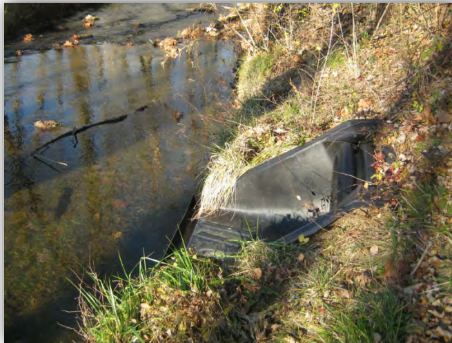
Figure 7. Regulated outfall within Jim Barnett Park limits. Outfall drains a Shenandoah University owned parking lot.
