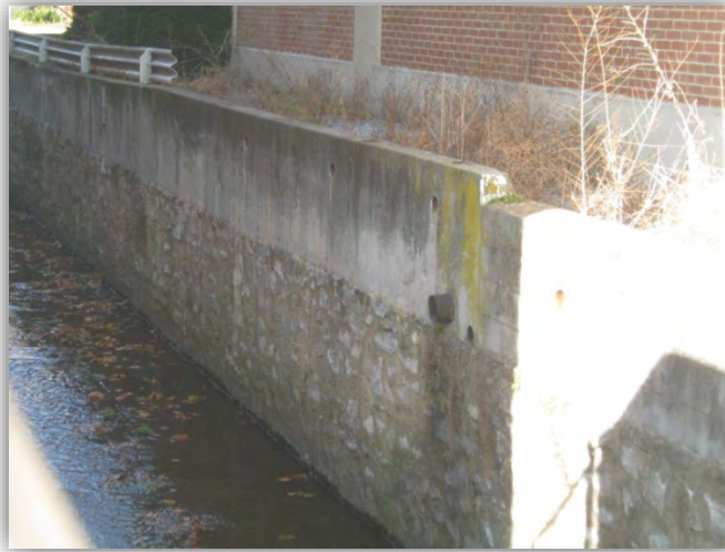
Figure 4. Court Square outfall locations (Roof Drains)
