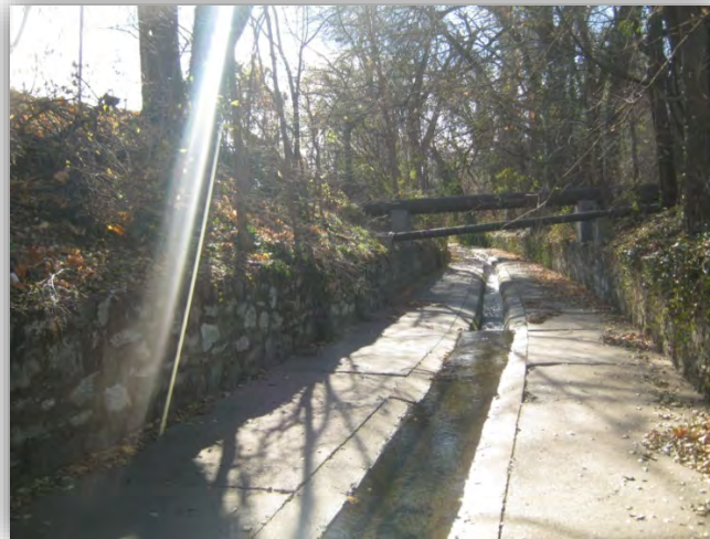
Figure 3. Concrete Channel (Actual City Owned Property)
