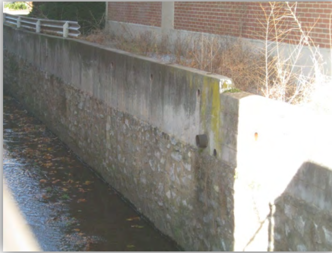
Figure 4. Court Square outfall locations (Roof Drains)
