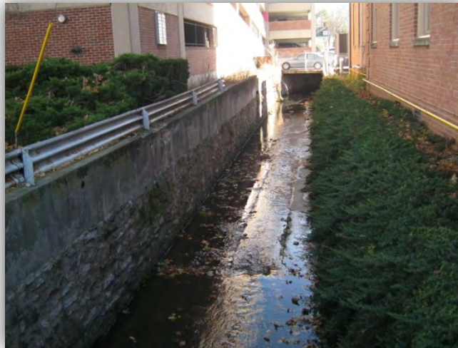
Figure 5. Stream running parallel and under Court Square Auto Park. Note: The outfalls discharge to the stream, but only drain the parking garage.
