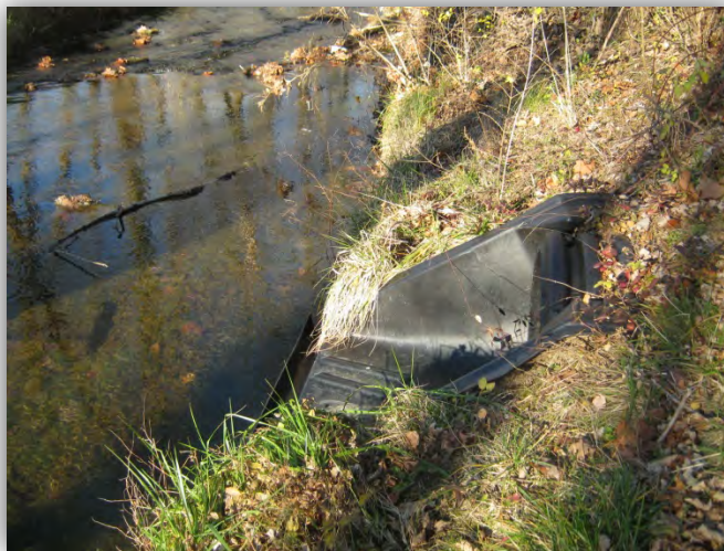
Figure 7. Regulated outfall within Jim Barnett Park limits. Outfall drains a Shenandoah University owned parking lot.
