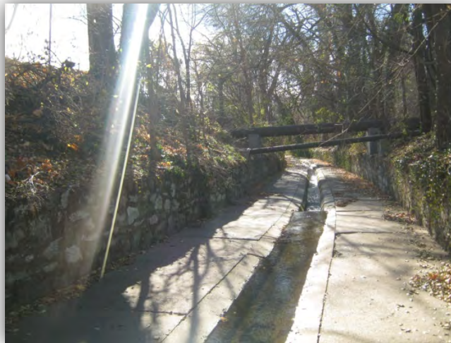
Figure 3. Concrete Channel (Actual City Owned Property)
