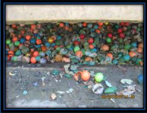
Paint balls in a catch basin
