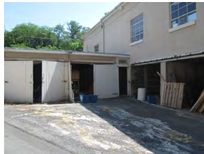
Photo 1.2 Title-City Yards Description-Road Paint Date Taken-6/20/2014
