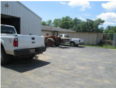
Photo 1.1 Title-Jim Barnett Park Maintenance Facility Description-Parking Area Date Taken-6/20/2014
