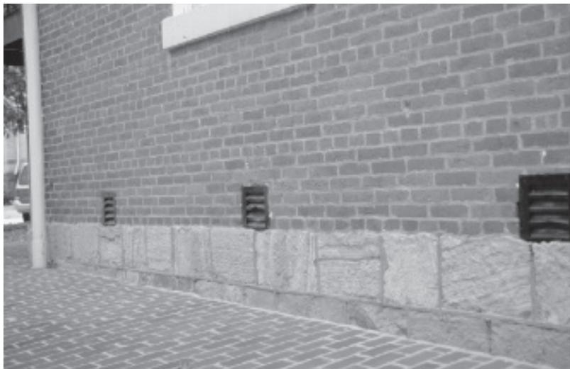
Foundation vents play an important role in keeping moisture from building up within the foundation.
